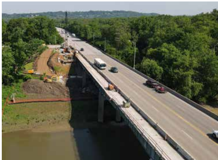
Looking west on Beechmont Levee, new trail added to south side of bridge.
