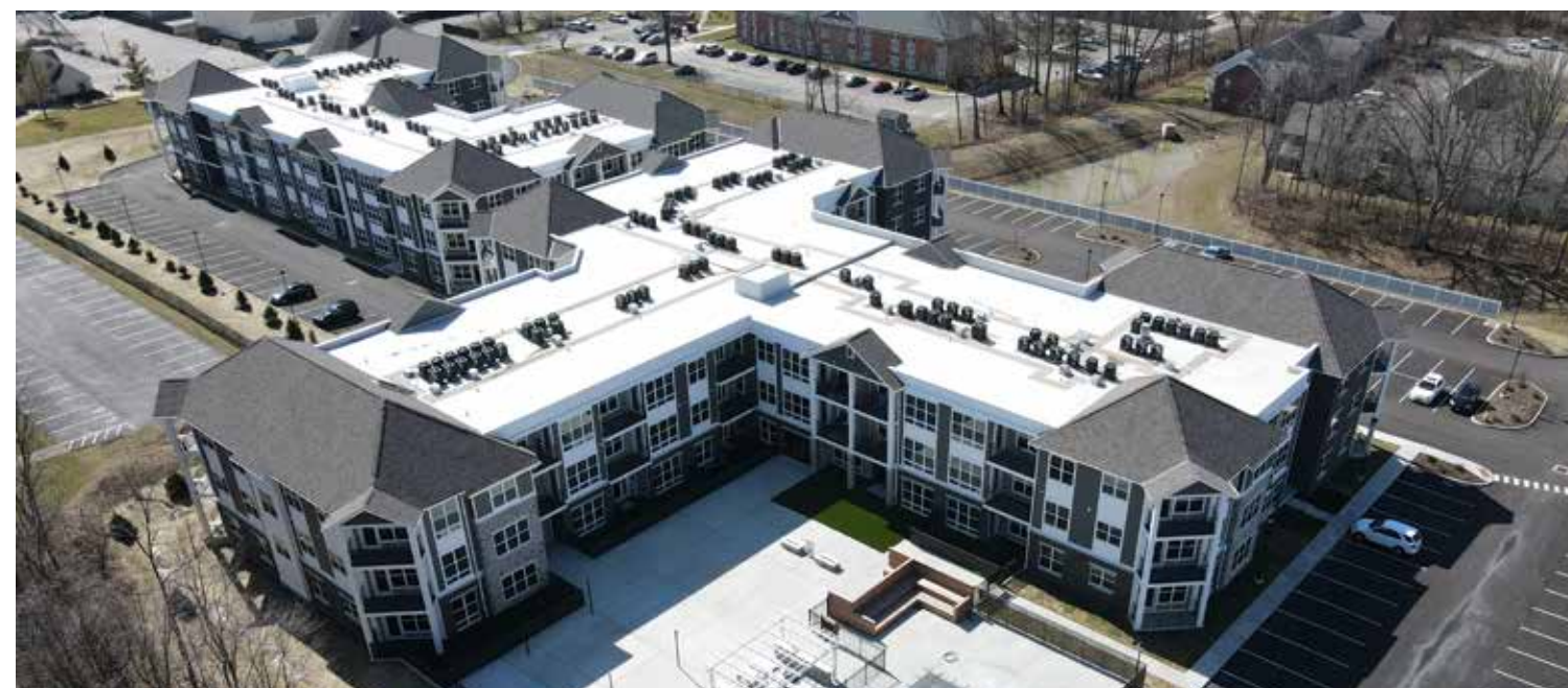
Stonegate Apartments - Phase 3
