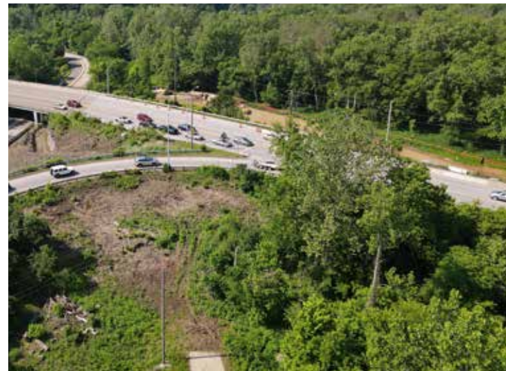
Current terminus of Little Miami Scenic Trail where tunnel will be built under the Ohio 32 ramp.
